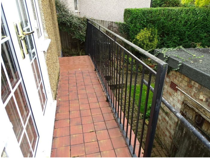
WALK ON BALCONY
