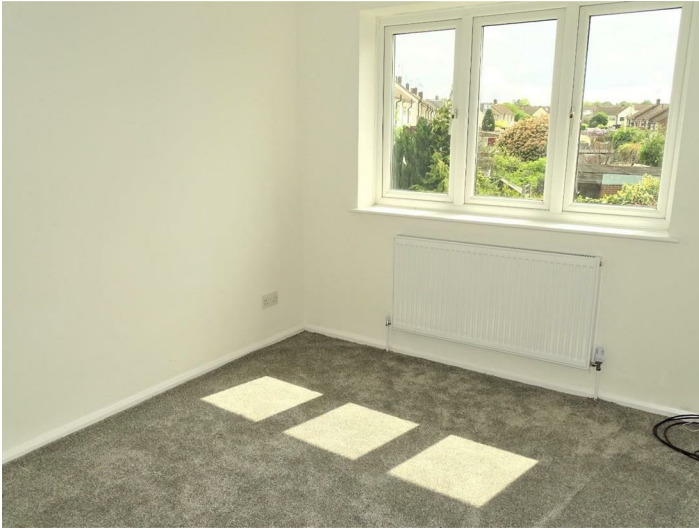
Radiator, upvc double glazed window to rear.
